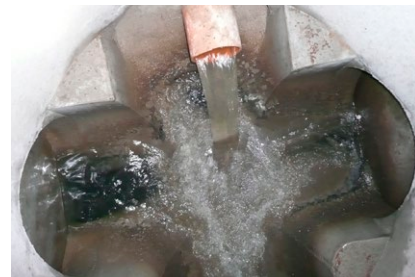
Oppumpningsbrønd for offerledning.
